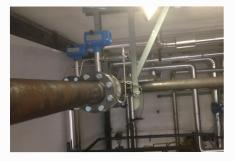
COMATE's VFM60MV vortex flow meter and TGF600 thermal mass flow meter are therefore used in the efficiency monitoring of steam boiler. The fuel could be natural gas or LNG, sometime it could biogas which is also produced in the factory from the food waste. The challenge is that the flow rate of those fuel consumption is always very small, so VFM60MV and TGF600 is the most cost efficient solution for a stable measurement of such small flow.
